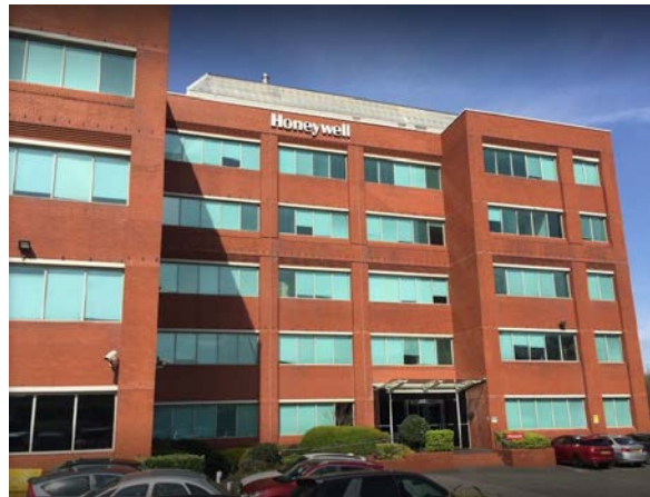
The Bracknell Training Facility
