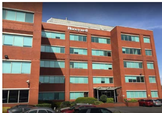
The Bracknell Training Facility
